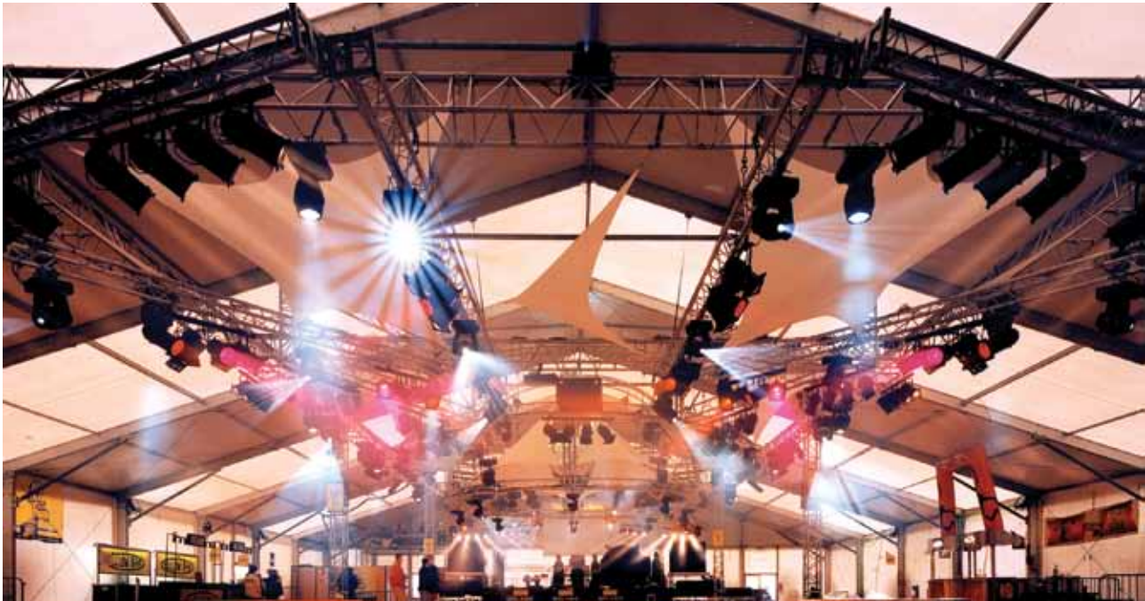
Photo: Prolyte. Project: Amusement park, Germany.
