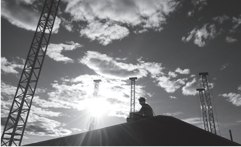
Photo: LT Roof, Aku's Factory, Finland
