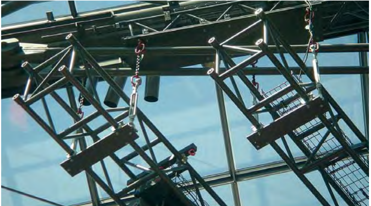
Photo: Prolyte. Project: Amusement park, Germany.
